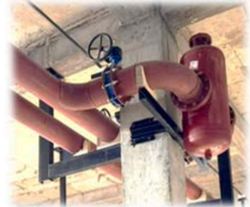
AIR SEPARATOR INSTALLATION
